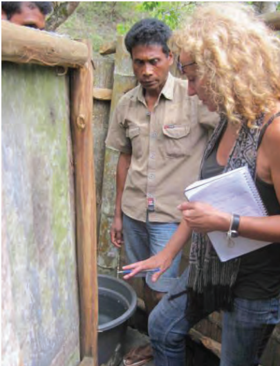
ENSURING QUALITY CONSTRUCTION: Monitoring of latrine improvements, Diric'un, Manatuto District, Timor-Leste.
